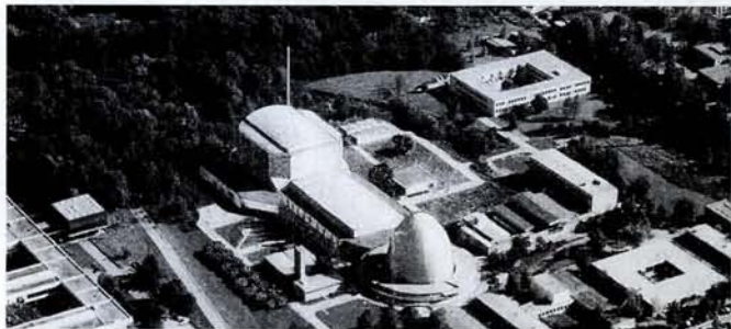
A photomontage showing a model of the new Forschungsreaktor München-II (FRM-II) behind the "egg" of the TU Munich's existing research reactor.
