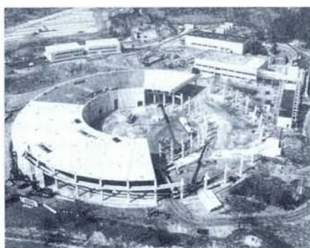
The ELETTRA synchrotron under construction near Trieste.
