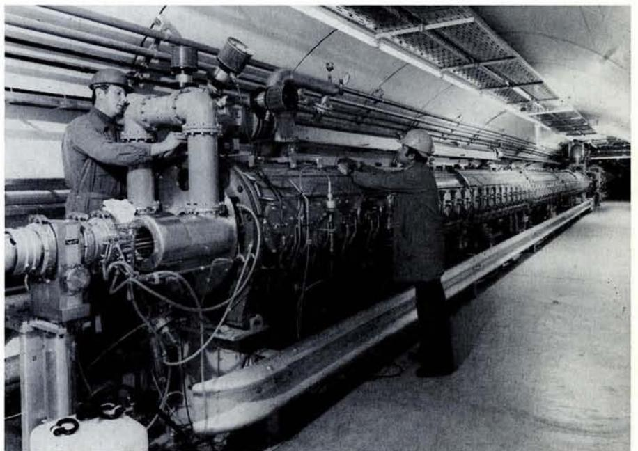
Fig. 1 One of the two accelerating cavities of the CERN SPS.
