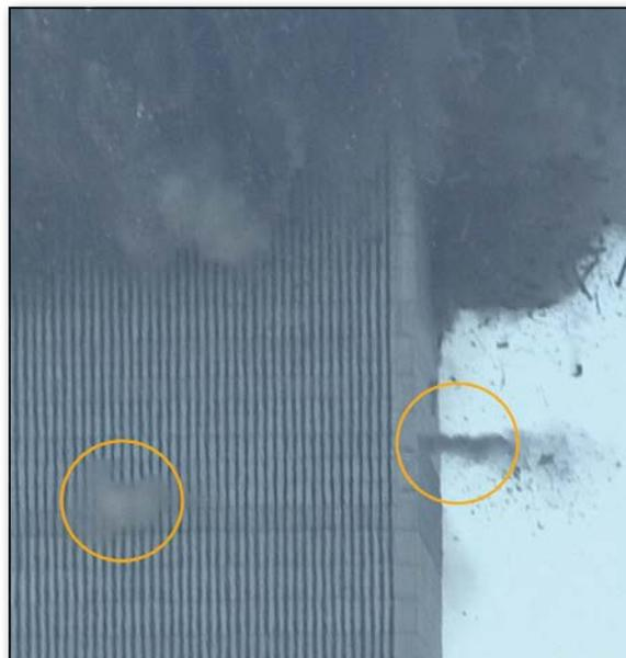
◀ FIG. 5: High-velocity bursts of debris, or “squibs,” were ejected from point-like sources in WTC 1 and WTC 2, as many as 20 to 30 stories below the collapse front (Source: Noah K. Murray).
